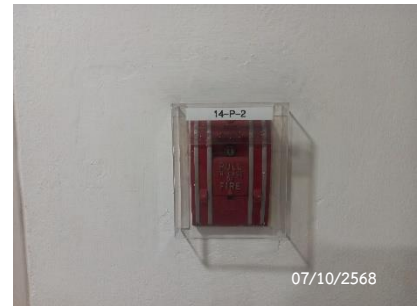
Fire Alarm Manual Station
