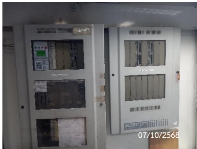
Fire Alarm Control Panel
